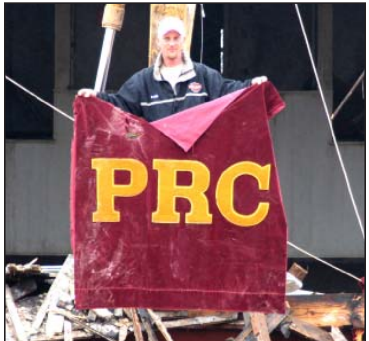
John Lee, a Holiday Construction Co. employee, holds the center section of the curtain that hung above the stage in Moody Hall auditorium. Lee rode up to the top of the stage in a track-hoe bucket to salvage the remnant of the old hall's history. The curtain will be conserved and placed in the museum.
