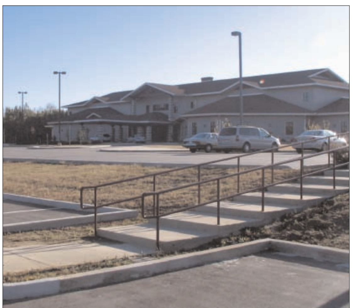
The Lowery Woodall Advanced Technology Center in Hattiesburg.
